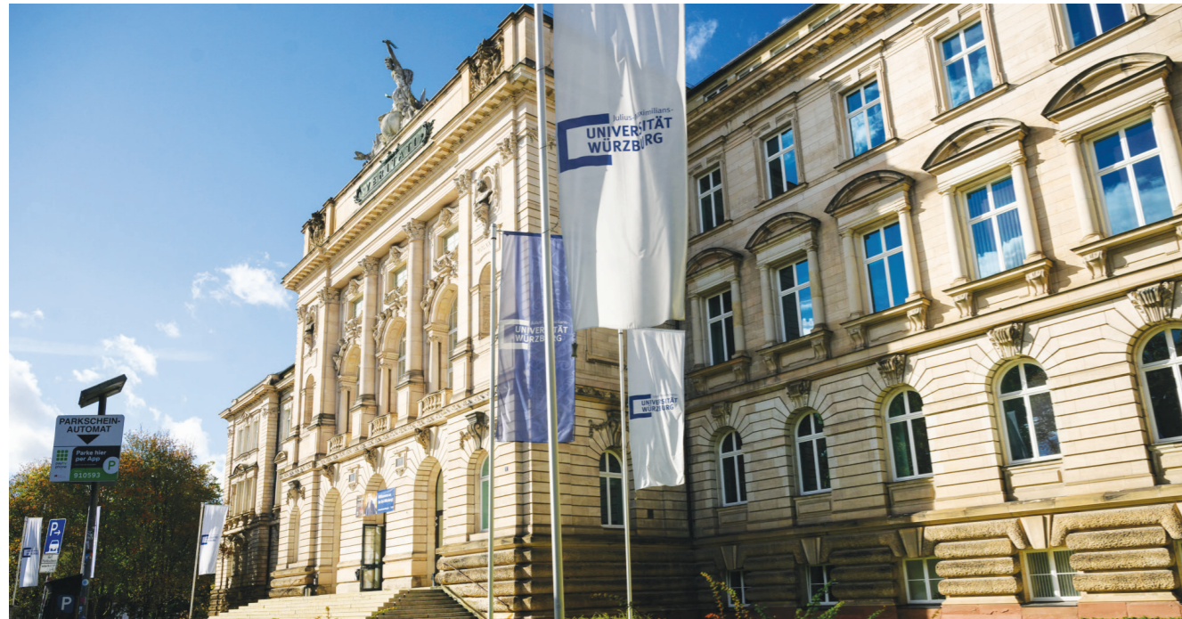
The Main Building of JMU
